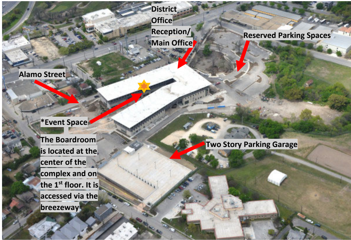
Alamo Colleges District Support Operations Complex
